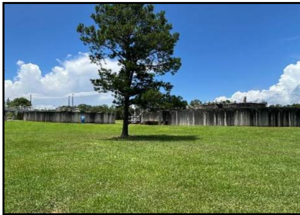
North of Area for Proposed Clarifier
