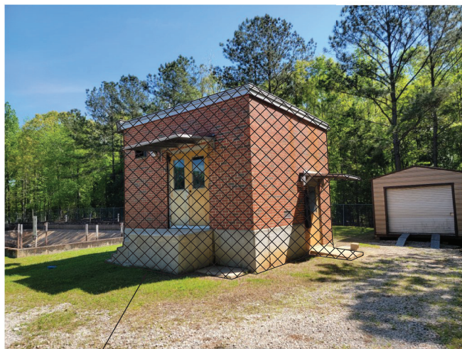
CARBON FEED BUILDING
