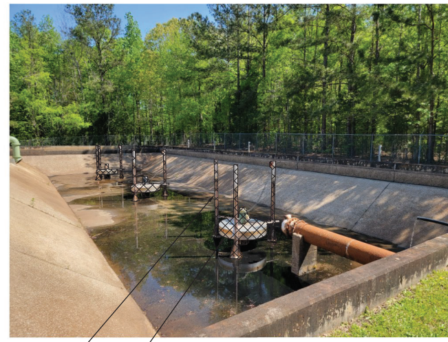
MOORING POLE (TYP) CARBON CONTACT BASIN MIXER (TYP)
