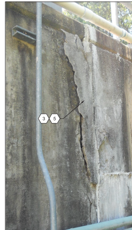
3 PHOTO VIEW (WEST BASINS 1&2 EXTERIOR WALL) NTS
